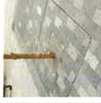
Stone Fence - metal railing 10/10/19
