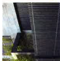
Stone Fence - metal railing 10/10/19
