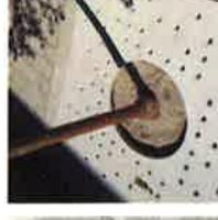
Stone Fence - metal railing 10/10/19
